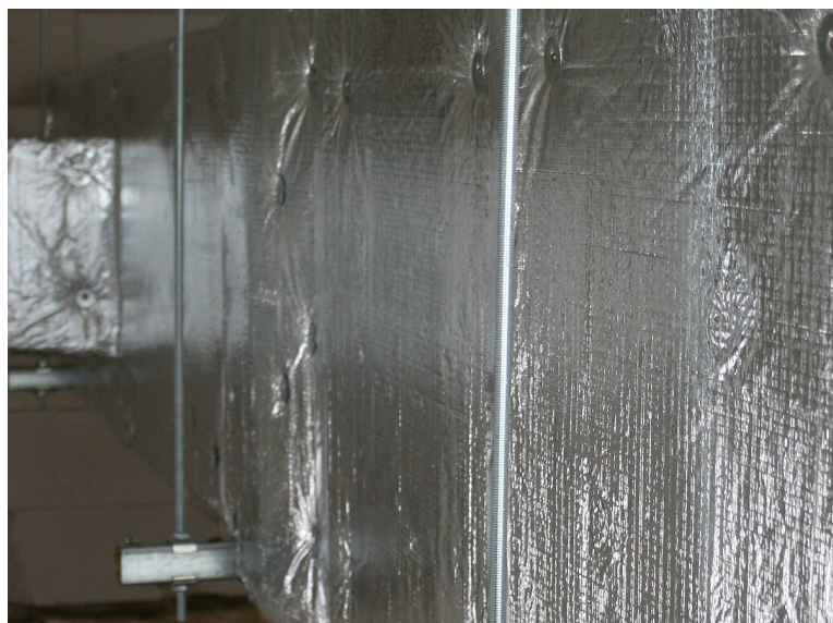
Fig. 1 - Example of Isover Cleantec G 100 application
