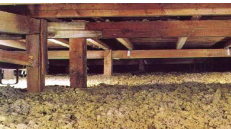
Fig. 5 - Blown insulation
