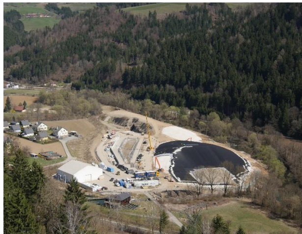
Figure 3. K20 contaminated site (as 28.3.2017) during remediation works
