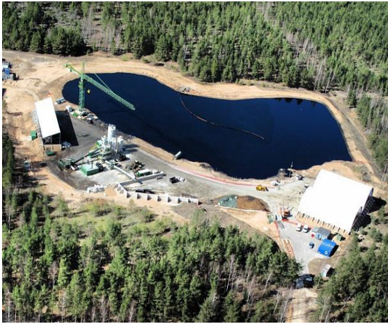
Fig. 2 Remediation of Southern acid tar pond [1]
