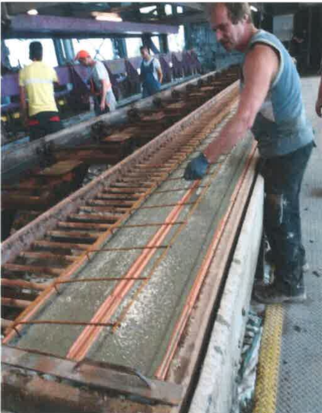
Photo 4 – Inserting steel reinforcement
