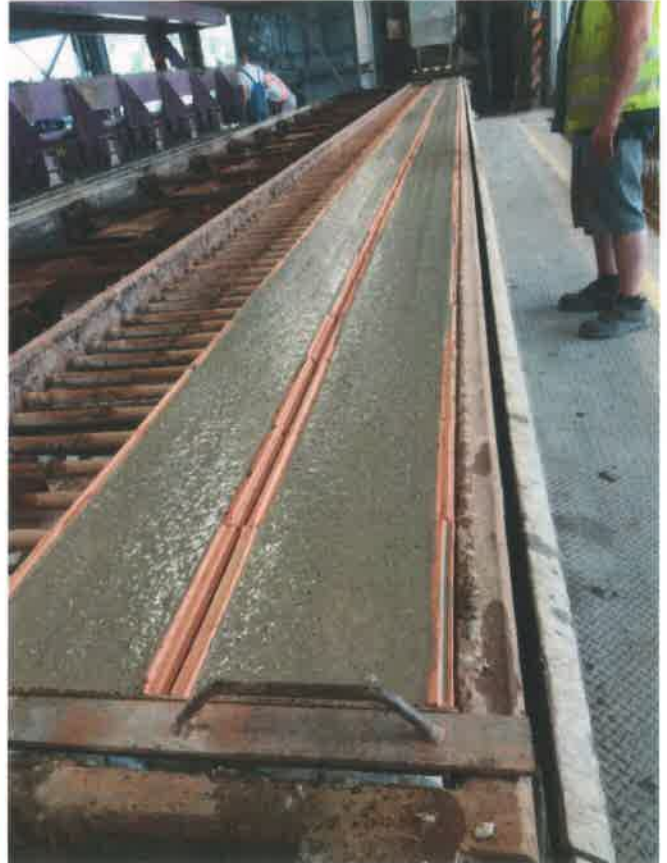
Photo 3 - U-shaped masonry units after concrete placement
