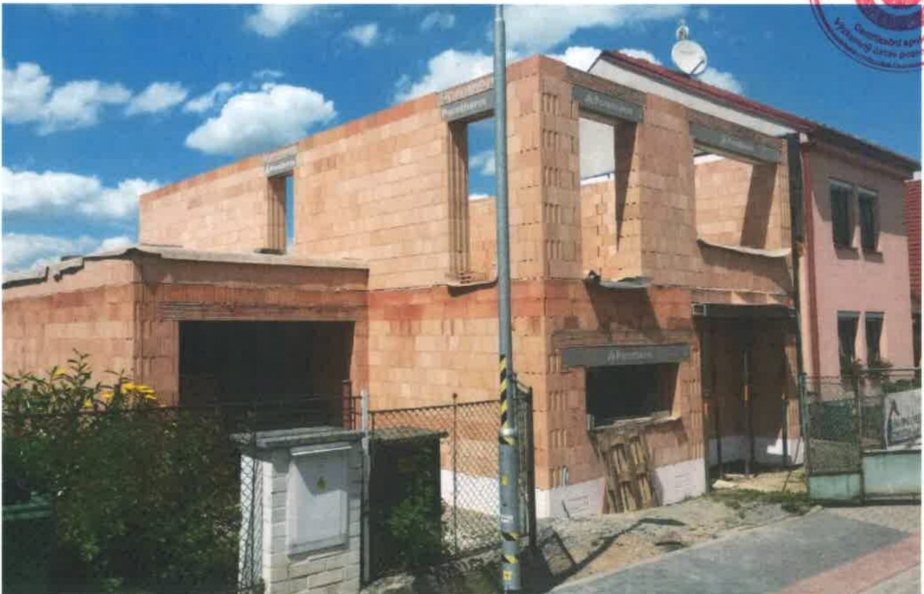
Photo 6 – Built-in KP Vario UNI lintels
