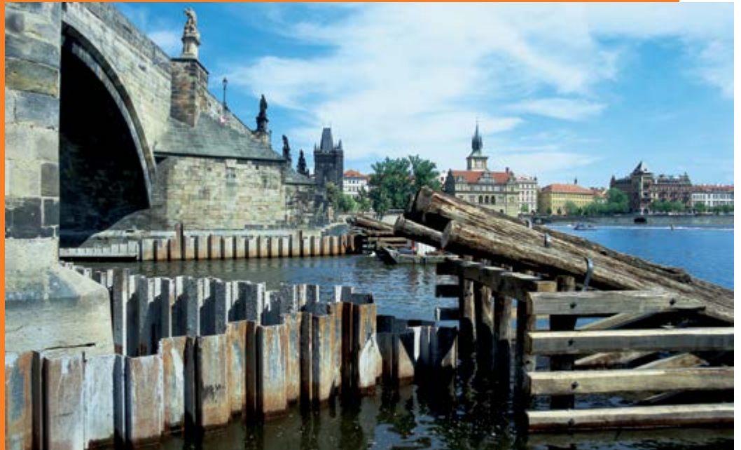
Pillars repairing of Charles bridge in Prague
